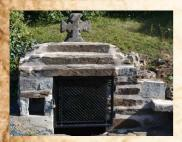
Dry stone masonry is a construction technique consisting of assembling, without any motar binder (cement, lime...), stones to mount a wall.
